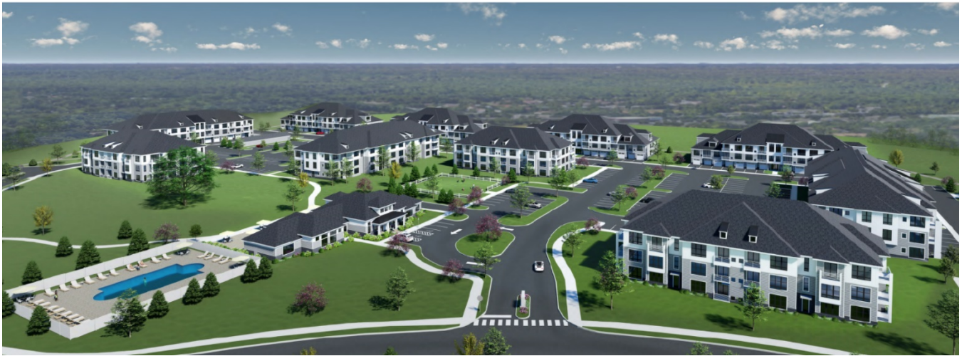
50-Acre Haddon Point Development currently under construction (600 residential units of apartments and townhouses)
