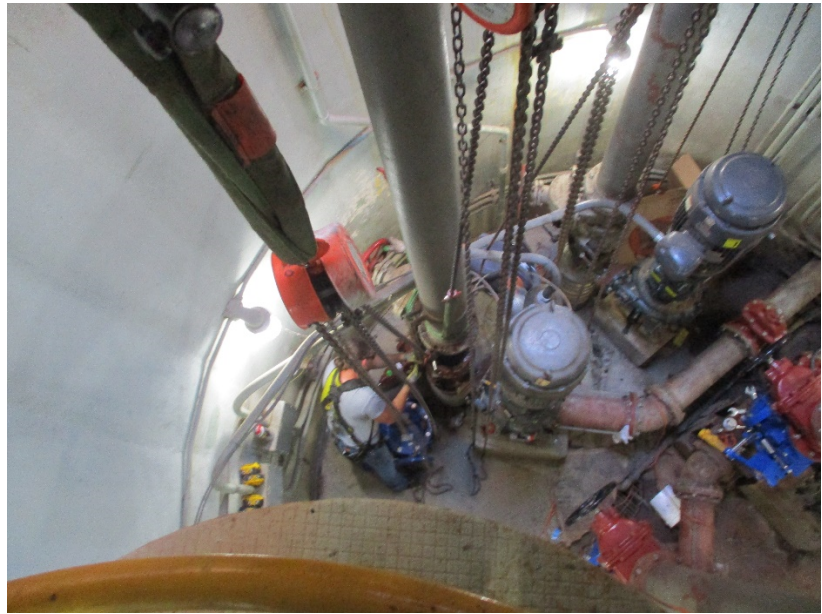
Replacing Valves in the Ramblewood Pump Station (the largest of the Authority's 41 pump stations)
