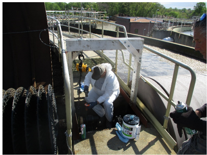
Repairs to Aerators & Replacement of over 700 Aeration Disks Orbal Oxidation Ditch Cell #2 Repairs
