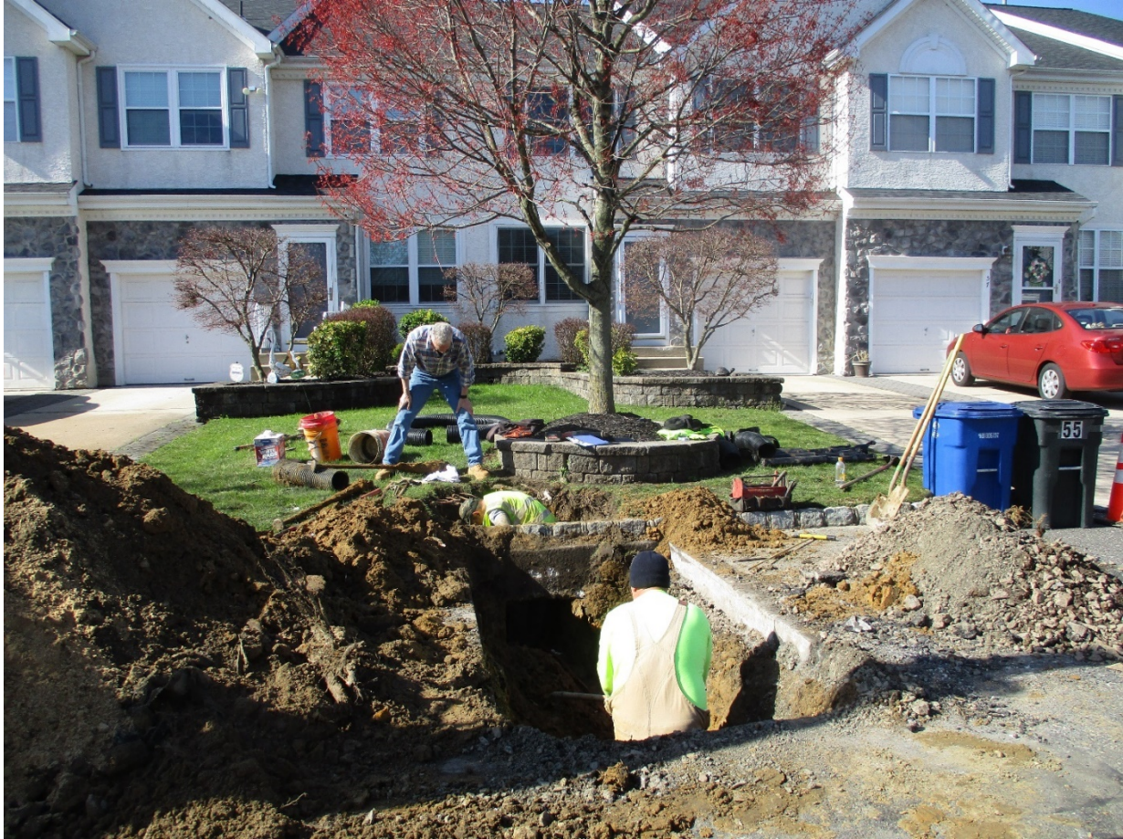
Installing Replacement Water Service Connections
