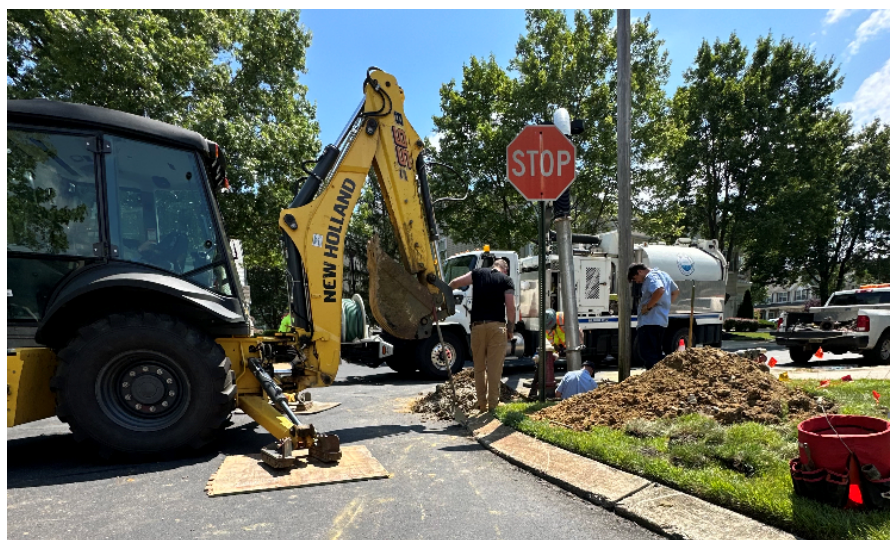
Replacement of a Fire Hydrant on Normandy Drive
