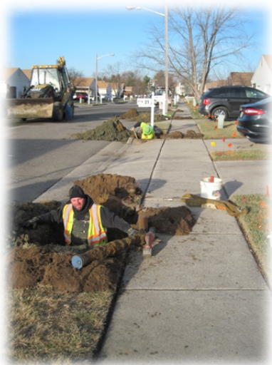
West Berwin Way Water Main Replacement – Curb Stop Excavation & Hydrant Installation
