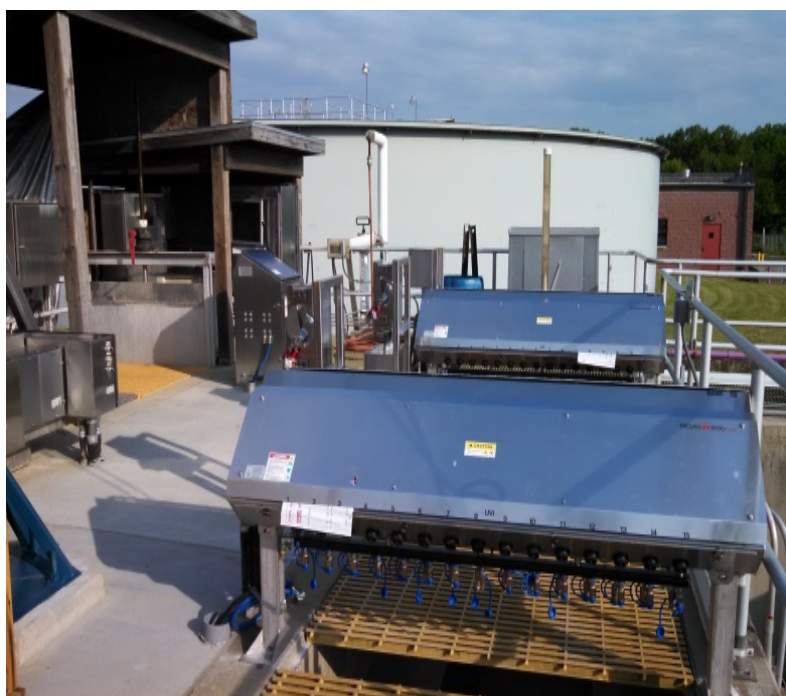
Hartford Road Water Pollution Control Facility – Ultra Violet Disinfection
