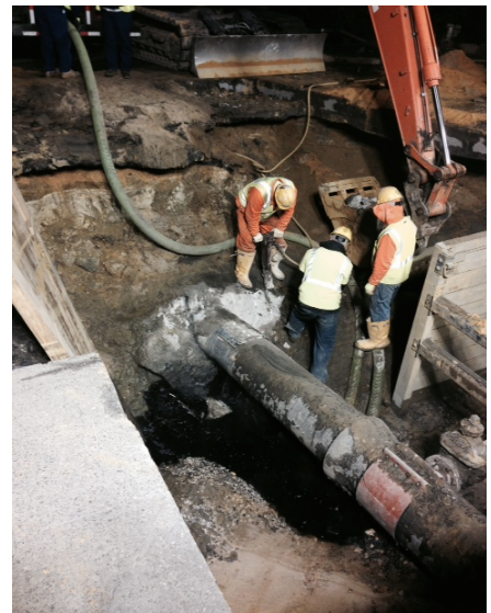
Union Mill Road Force main repair
