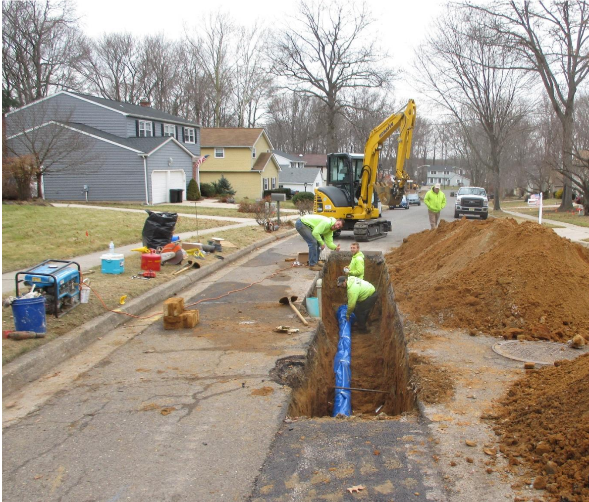
Section of new water main wrapped in protective plastic
