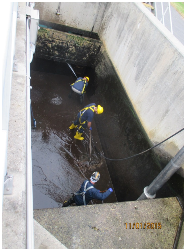
Working on the Hartford Rd WPCF UV Disinfection Tank Gate
