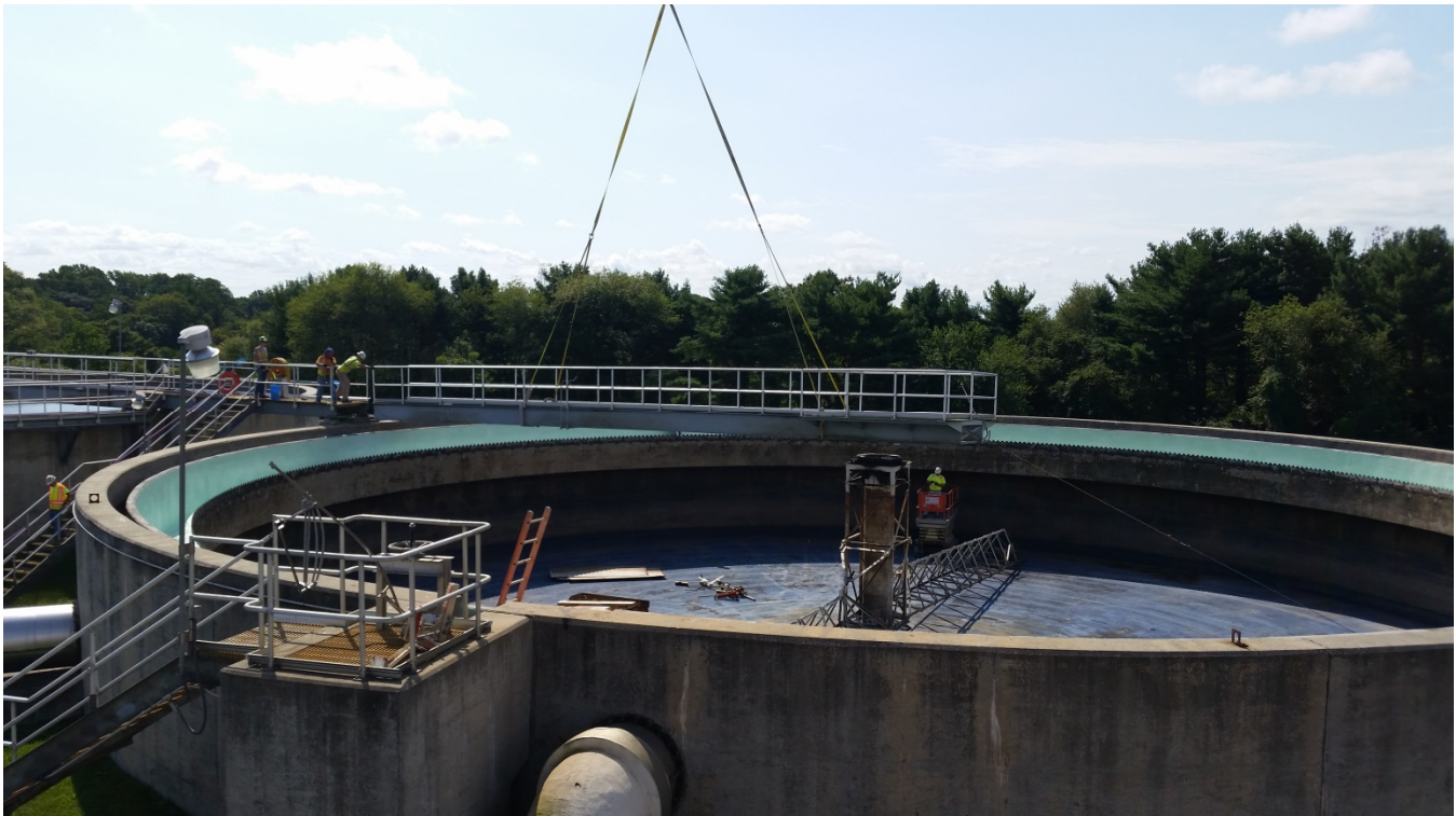
A crane removes part of the Secondary Clarifier bridge as part of the $ 506,025 rehabilitation project which began in FY15 and was completed in FY16
