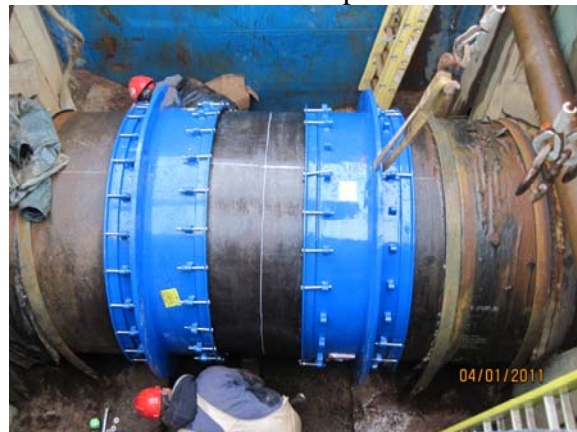
Sleeve and repair clamps in place
