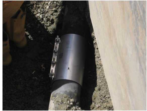
Forcemain in Stonegate - Repaired
