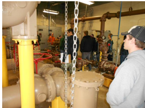
RAS/WAS pump room at sewer plant
