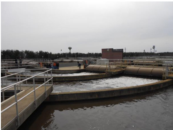
Orbal tank at sewer plant
