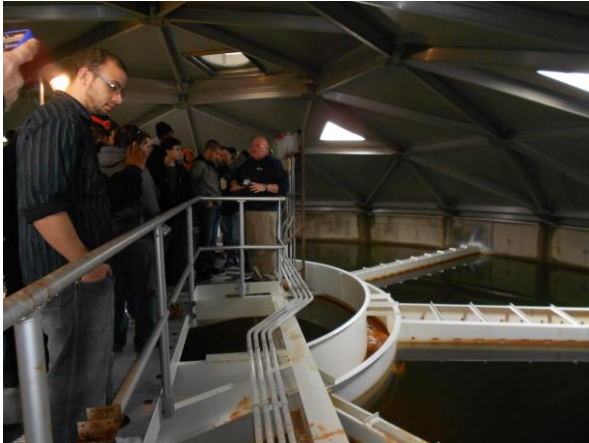
Clarifier at the water plant
