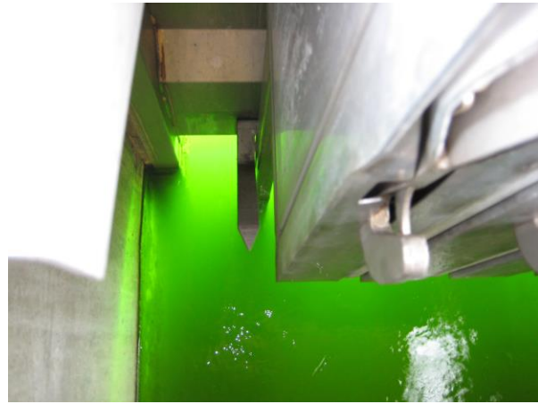
Wastewater passing through UV system
