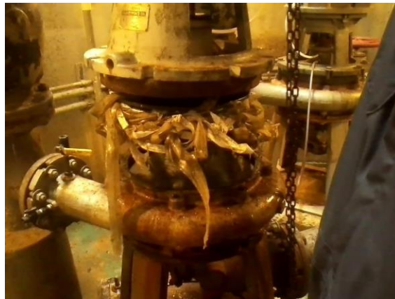
Ramblewood PS – Slip Lining from Ramblewood Parkway Came Off
