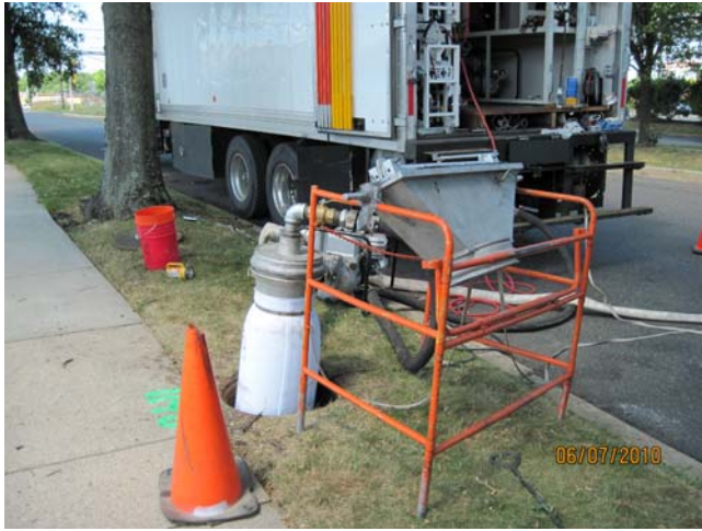
1 st Section of Liner
