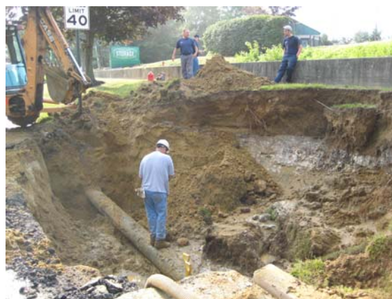
Locating the damaged main
