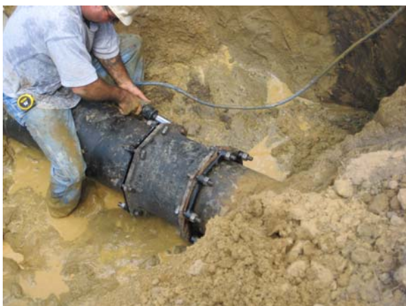
Installation of the replacement main
