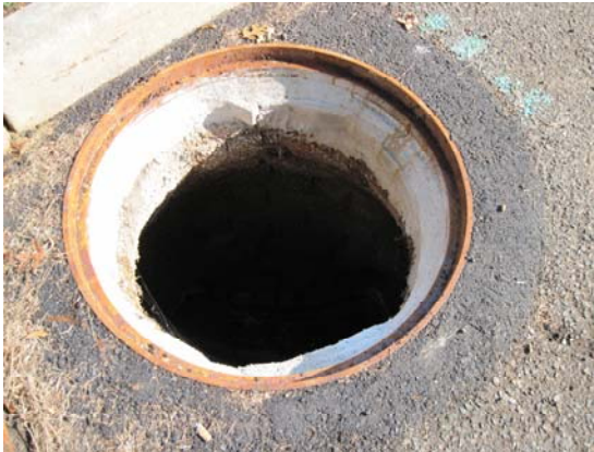
MH # 1147 before grouting
