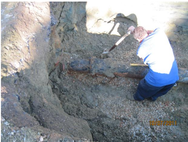
Original corroded water main (to be replaced)
