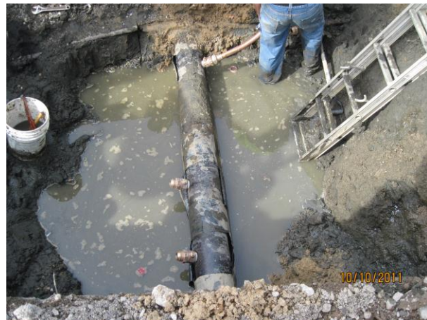
Tapping residential service lines to the new main
