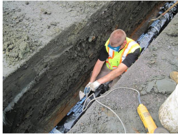
Welding of sacrificial anode onto new pipe encased in plastic (2 forms of corrosion protection)
