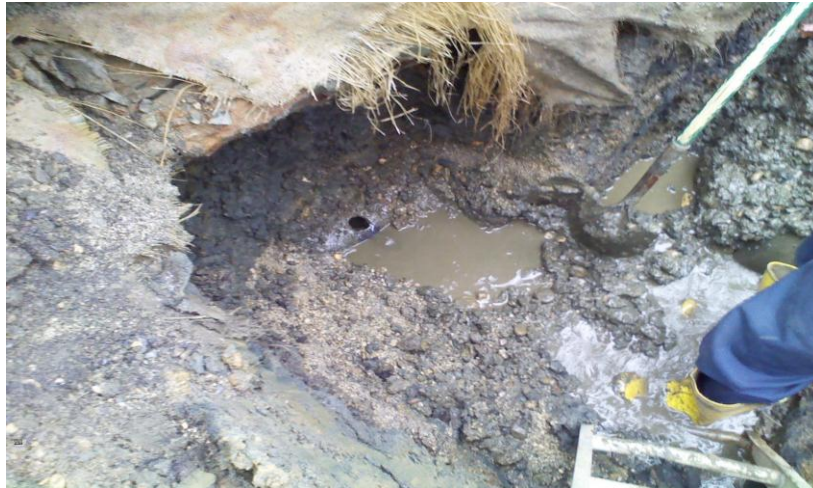
Watermain Millstream Drive & Windsor Lane Found hole in watermain from corrosion
