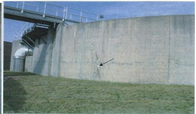
Clarifier #2, exterior with efflorescence
