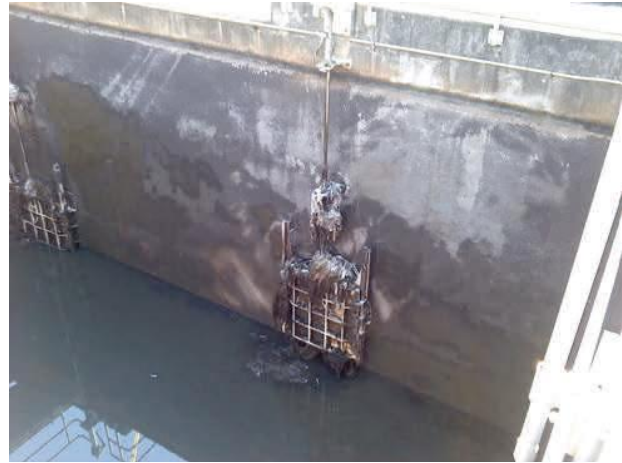
Orbal Cell #1 interior, sluice gates
