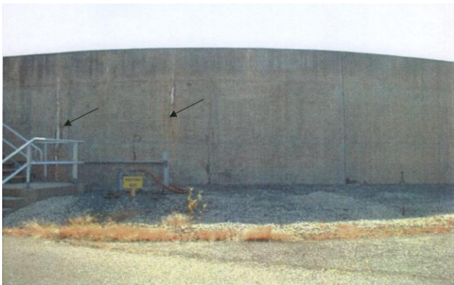
Orbal exterior with efflorescence
