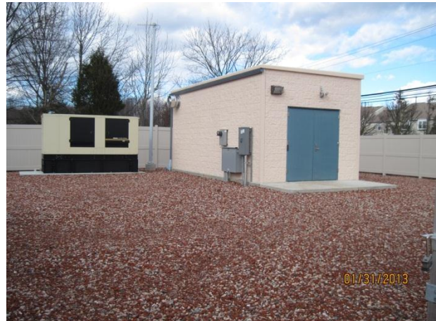
New well bldg. with permanent standby diesel generator
