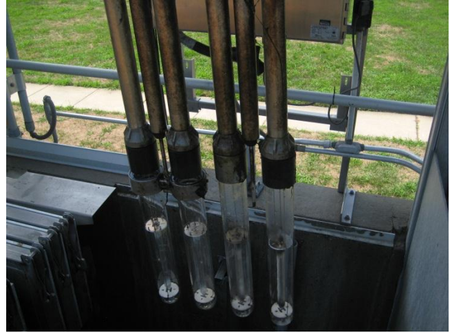
A cleaned UV module arm
